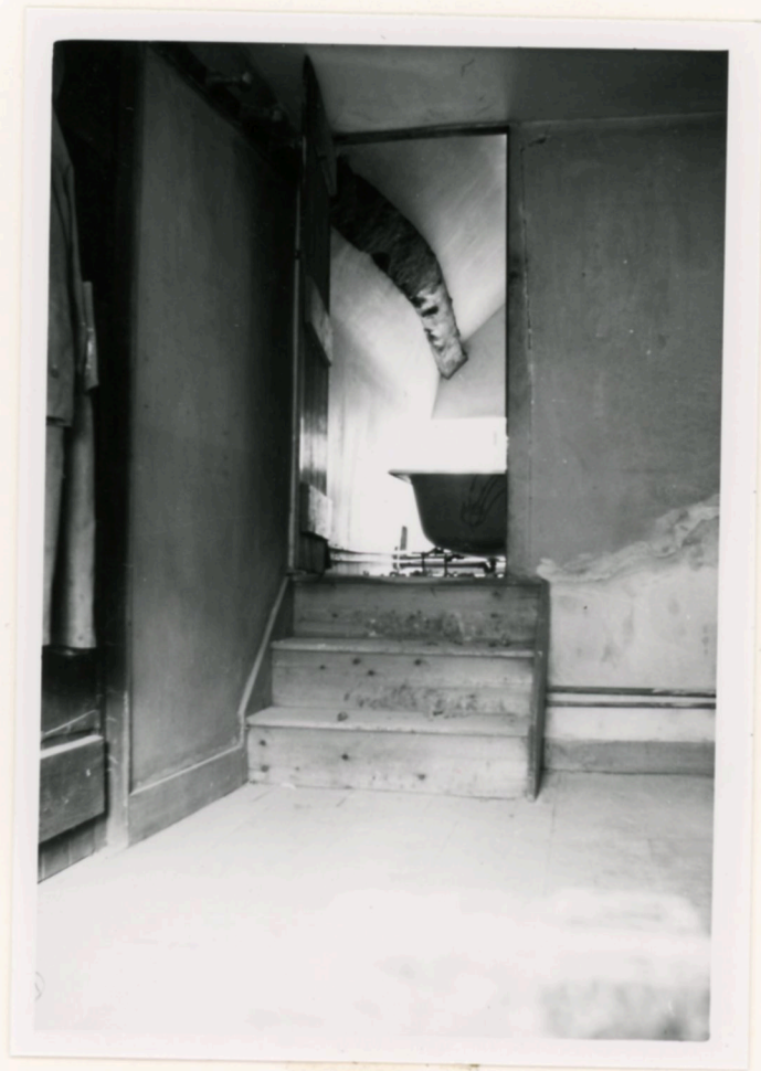
Steps up to tallat (now bathroom) above kitchen
