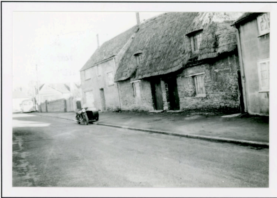
Unrestored, early 1963. Two doors, small workroom window and crooked lintel to blocked in window. Low irregular thatch.
