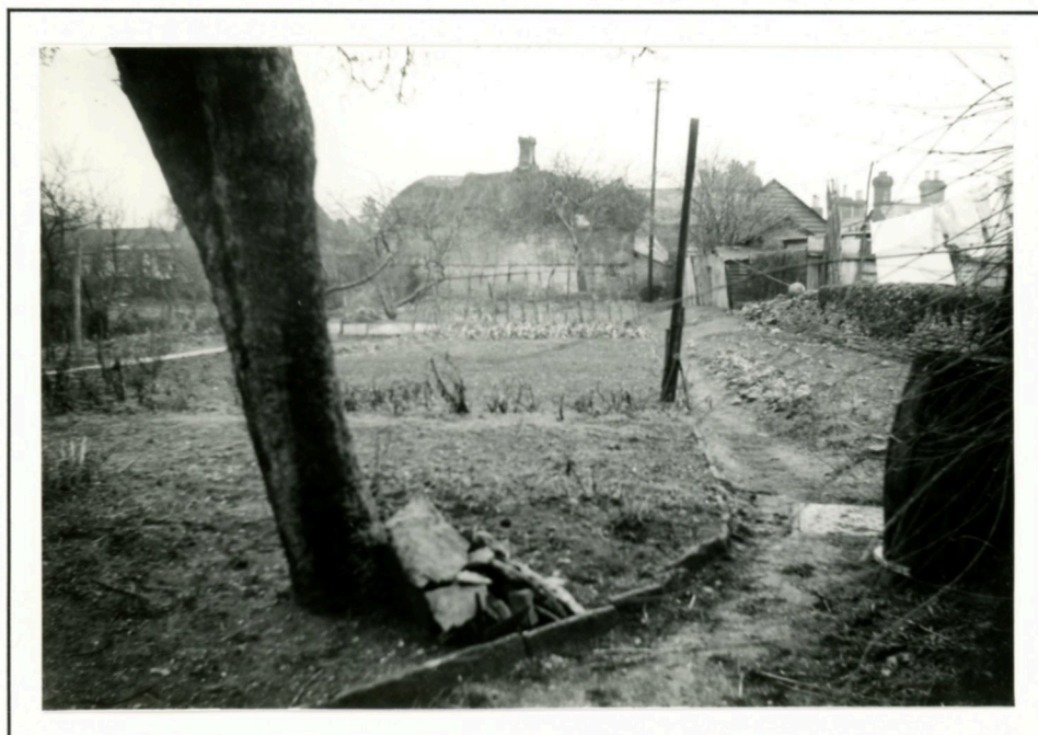
Looking up the garden: Plaster's shed on right. Derelict 'barn' with chimney behind dying appletree, centre. (1963).
