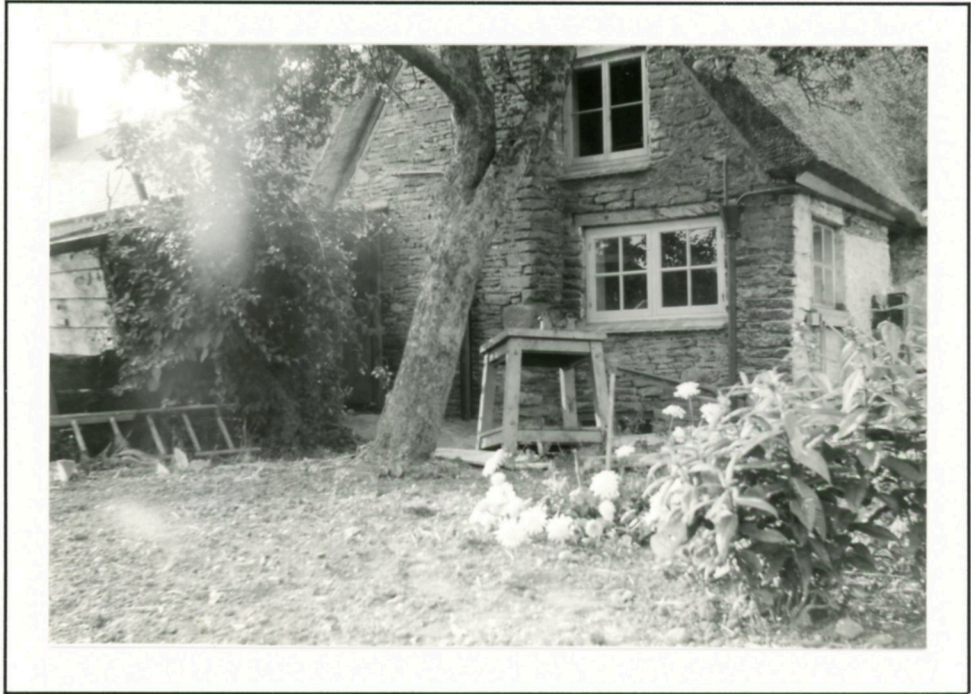
Same windows restored to original size and reframed. Shelter to back doors removed (whitewash under). Sunroom not yet built but plumbing installed (1963).
