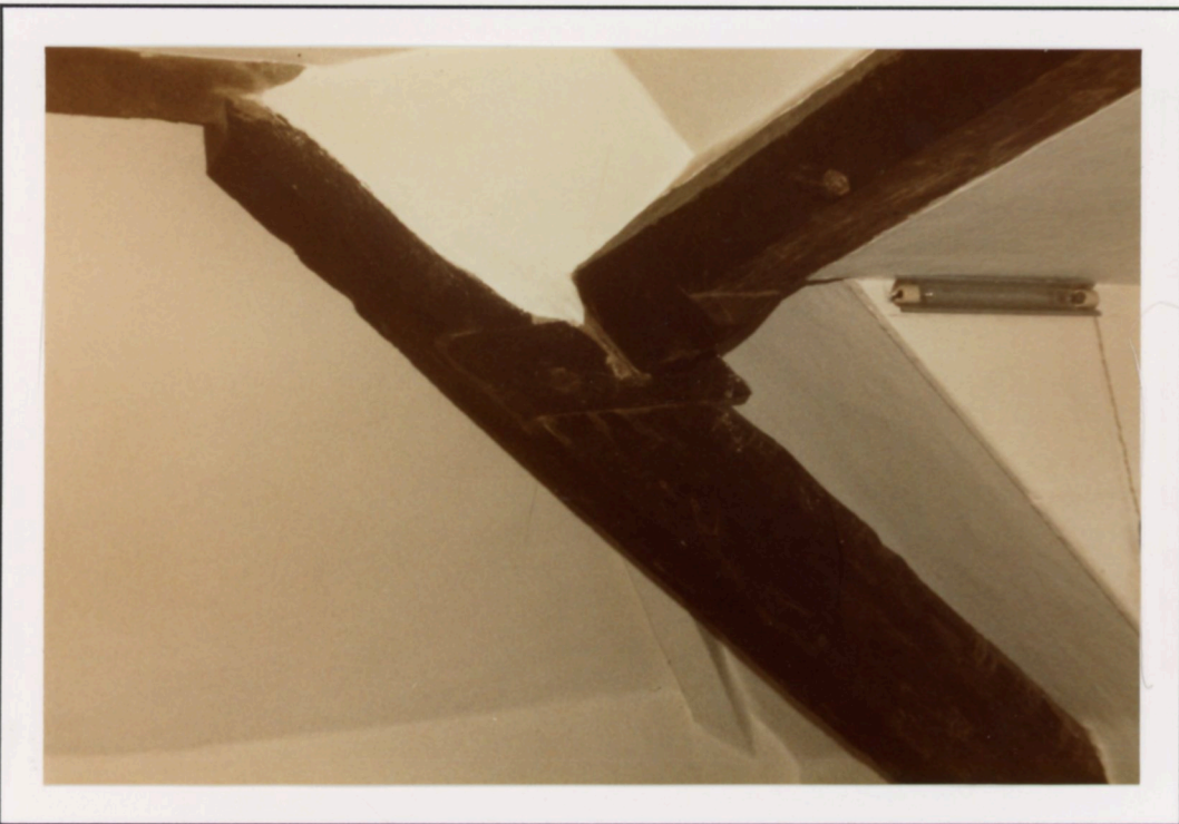
Corner diagonal beam in second bedroom, free of the roof structure: put there possibly because the window gable beam was not long enough to reach the opposite wall. Even then the joint seems to have been botched with an inserted cradle.
