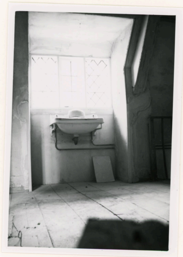
Washbasin installed in south recess in main bedroom
