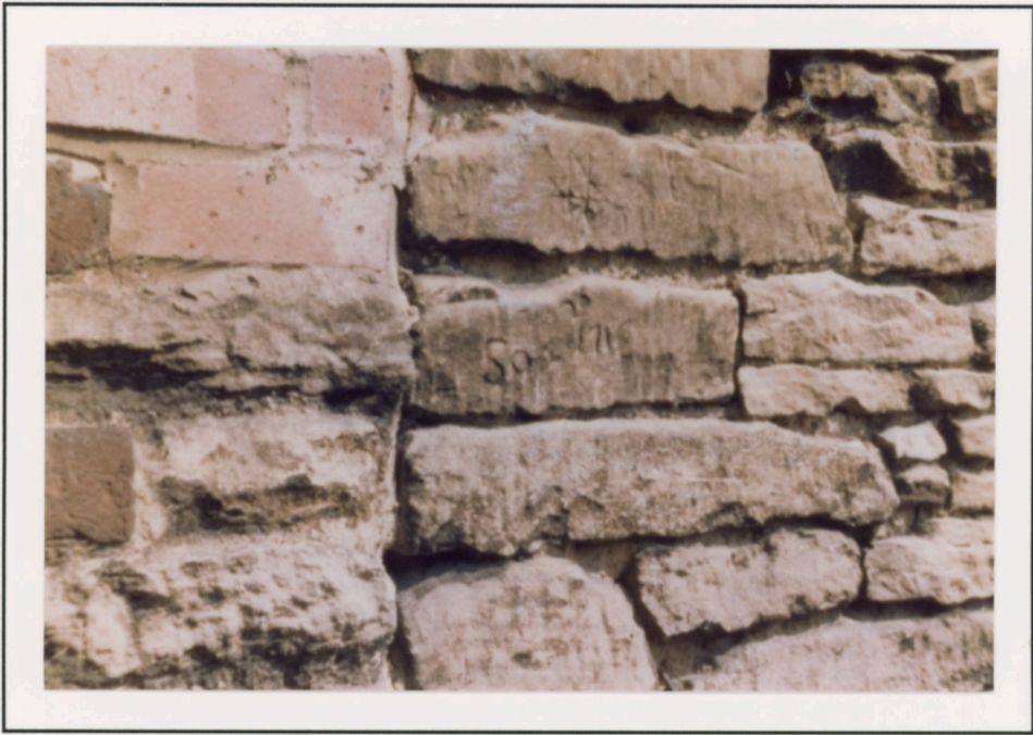
Older work with modern chimney insertion
