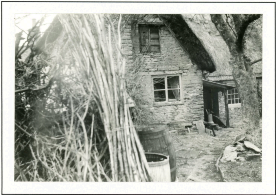
South kitchen window and that to the tallat above had both been reduced in size. Note corrugated shelter to back doors. Pigstye was in tangle on extreme left. (1963).
