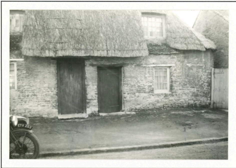
Original: Two front doors, one shorter. Small window under long lintel. Note Stonesfield slating to upstairs windows. (1963).
