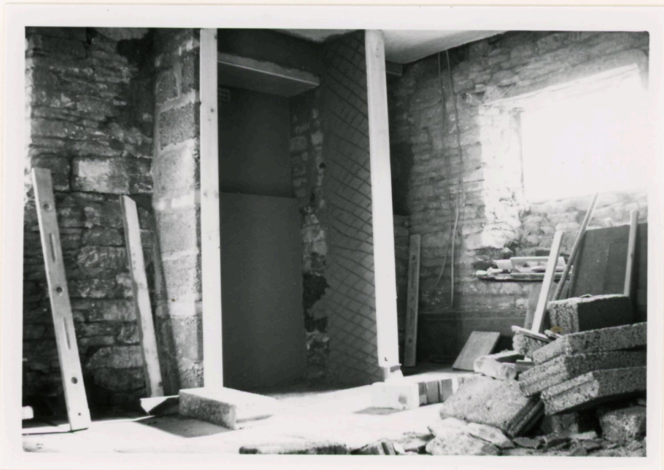
Kitchen: S.W. corner (see pic. on right). Overmantel to kitchen removed, food cupboard being constructed
