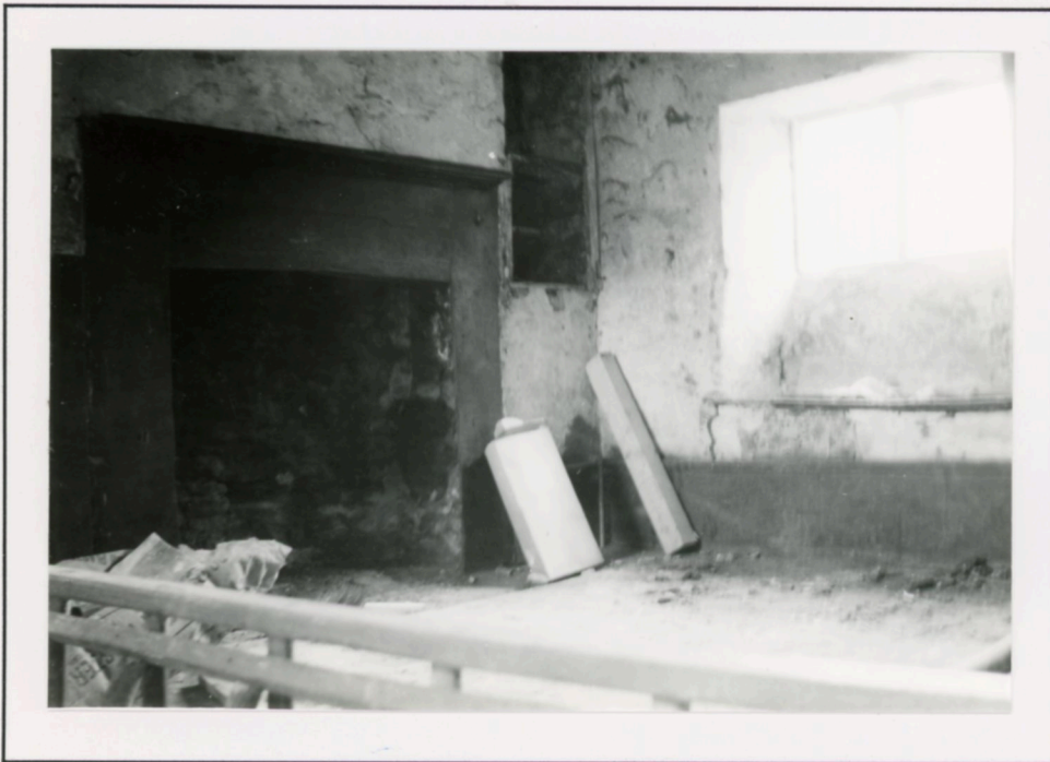
Kitchen: South west corner. Kitchen range has been removed. Over mantel remains pro tem. Deep alcove in extended external chimney breast, centre. (1963).
