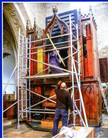
Another large pipe coming out
