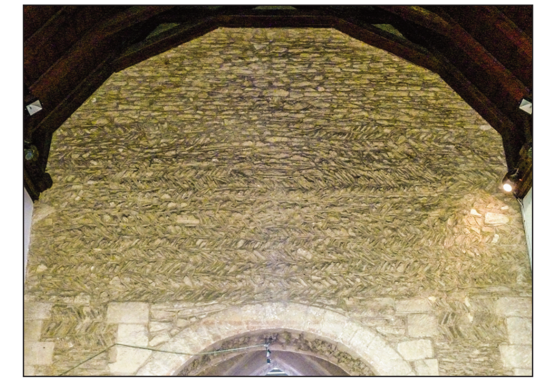
Herringbone masonry
