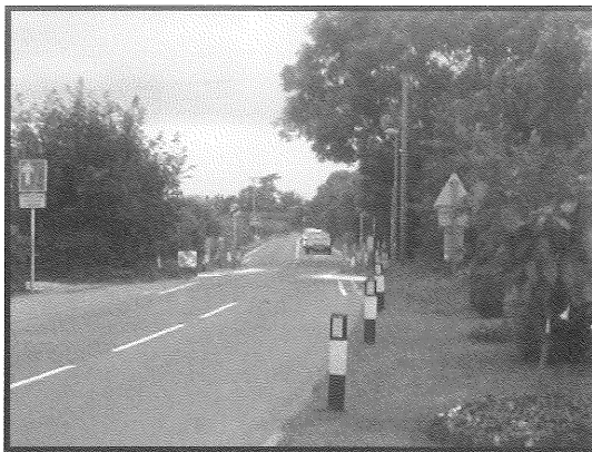
The Buildout/Chicane at Station Road Physical Barrier Slows down car in both directions
