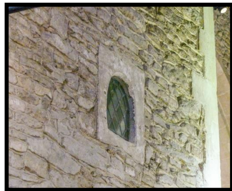
Window in N wall of stair turret
