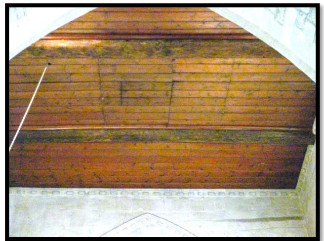
Wooden ceiling, the floor of ringing chamber
