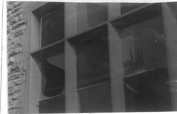
AIR - CONDITIONING AT THE OLD SCHOOL photo: Richard Yapp
