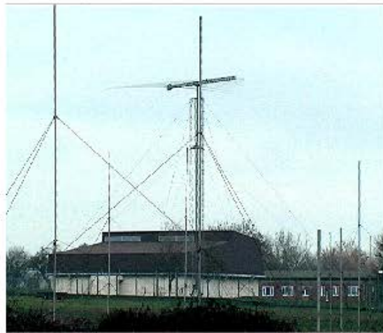
The L P in the background. With the Bunker built post '69. The Royal Signals Hall to the right. Vertical antennae for RDF foreground.
