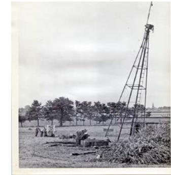
Tower removed from Windmill Farm, Bampton for use as aerial mast
