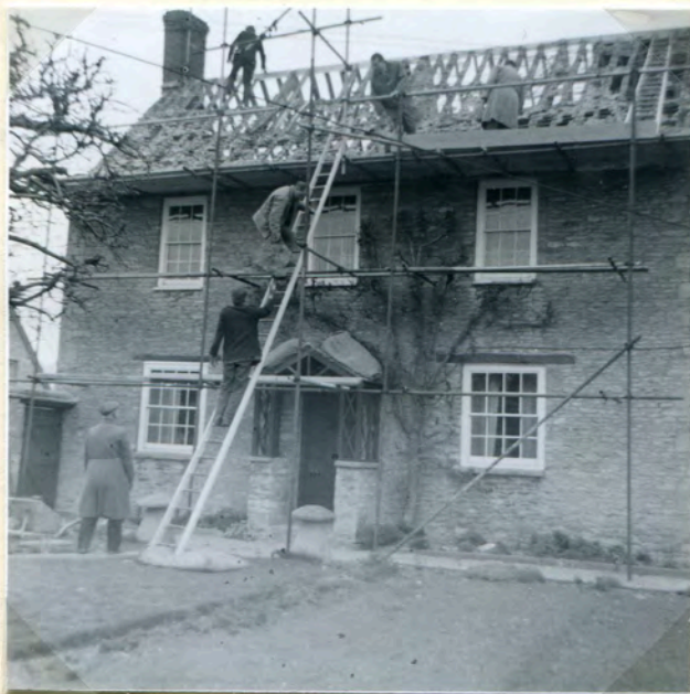
Sandfords House Re-roofing with original slates
