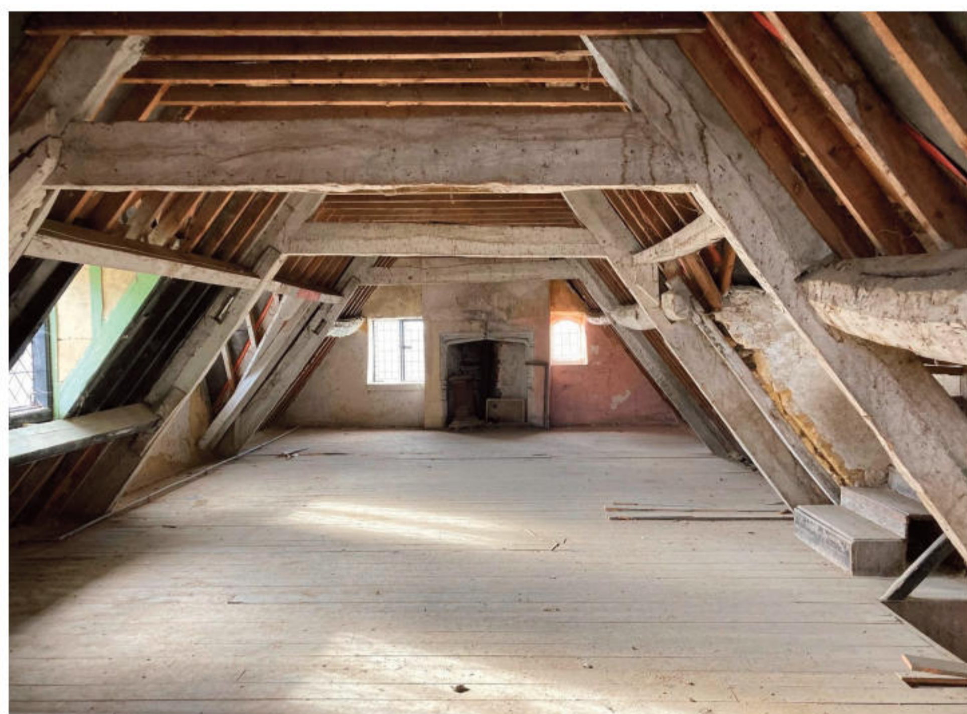
The upstairs space before the restoration started
