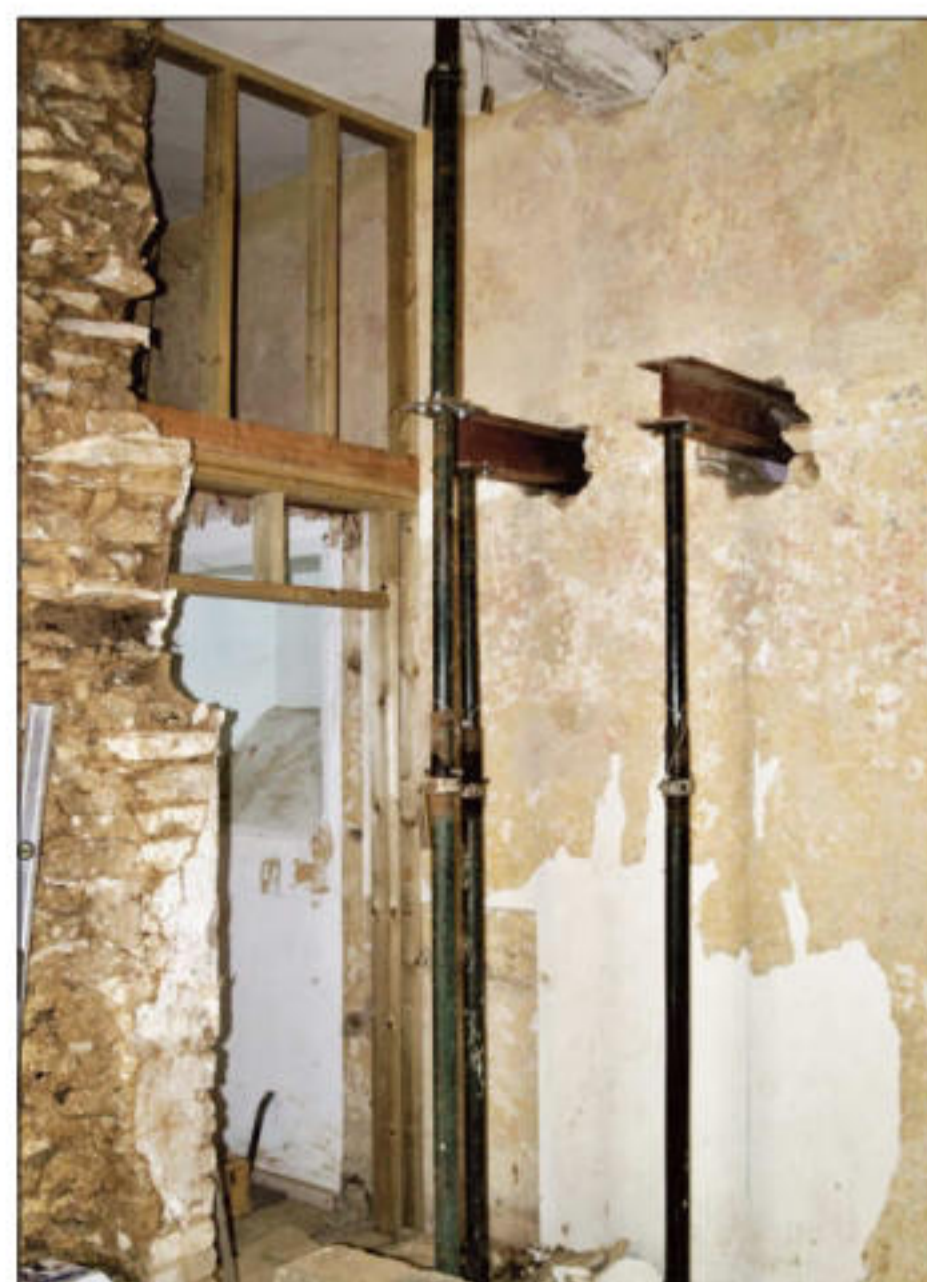
Pinning before cutting out new library doorway
