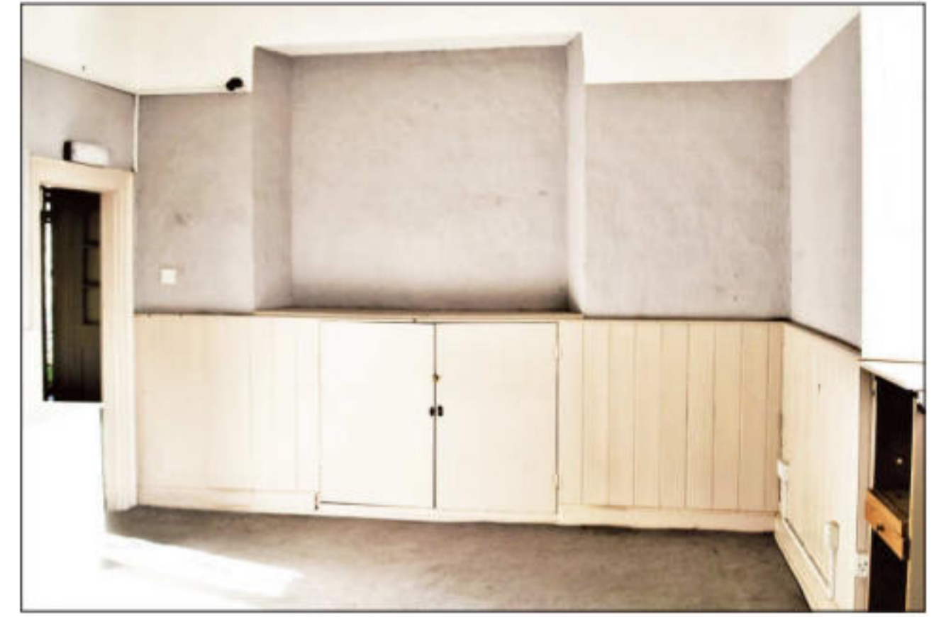
Vesey Room before work began
