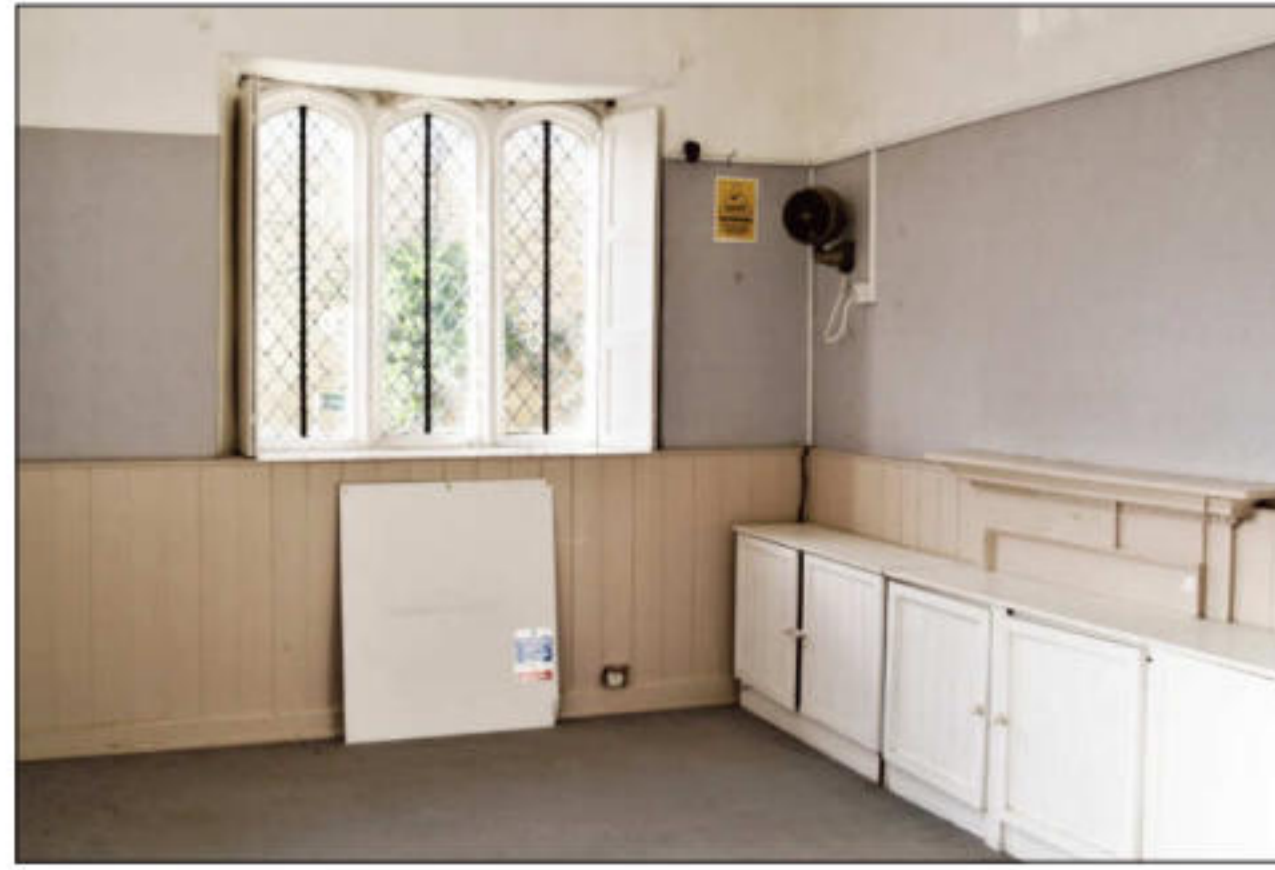
Vesey Room before work began
