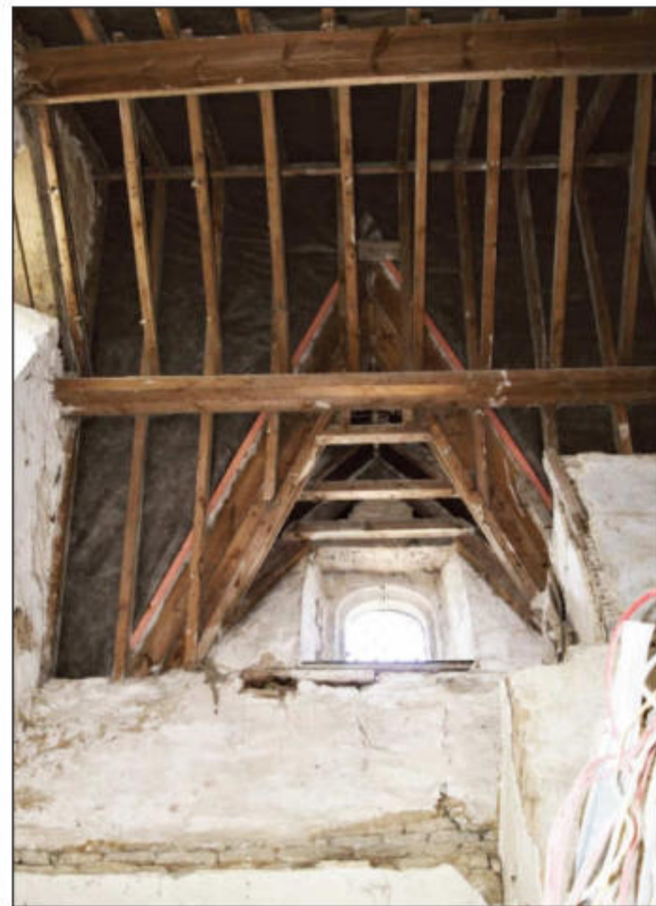
Roof structure after ceiling removed
