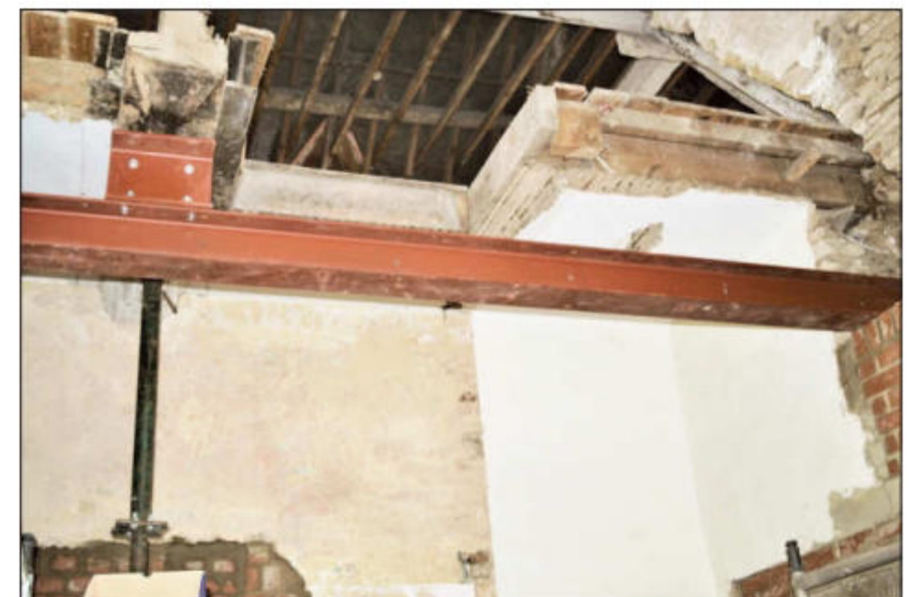
Steel beam installation
