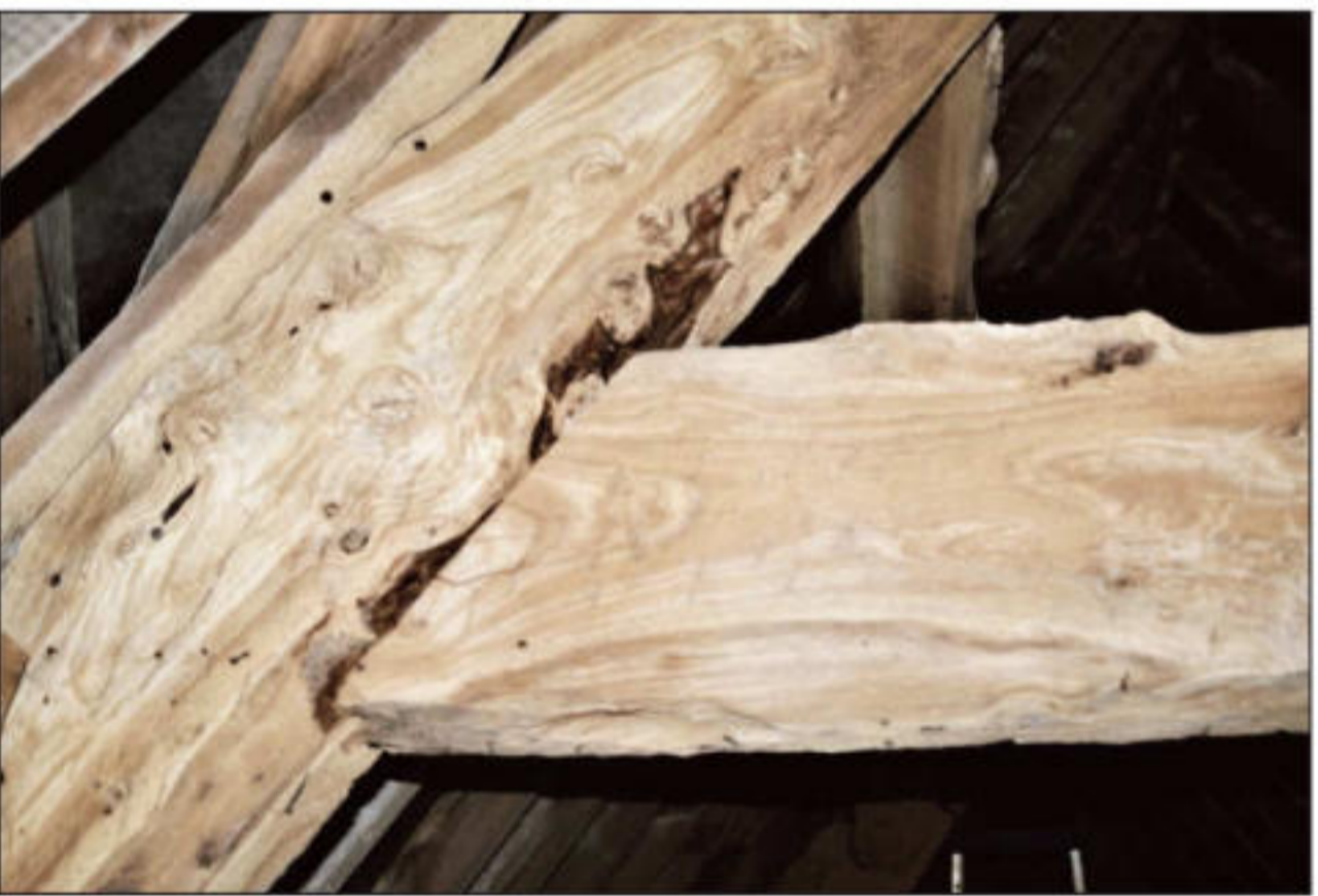
Grit blasted roof truss joint
