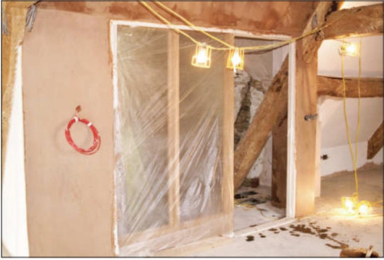
Glazed screen installation
