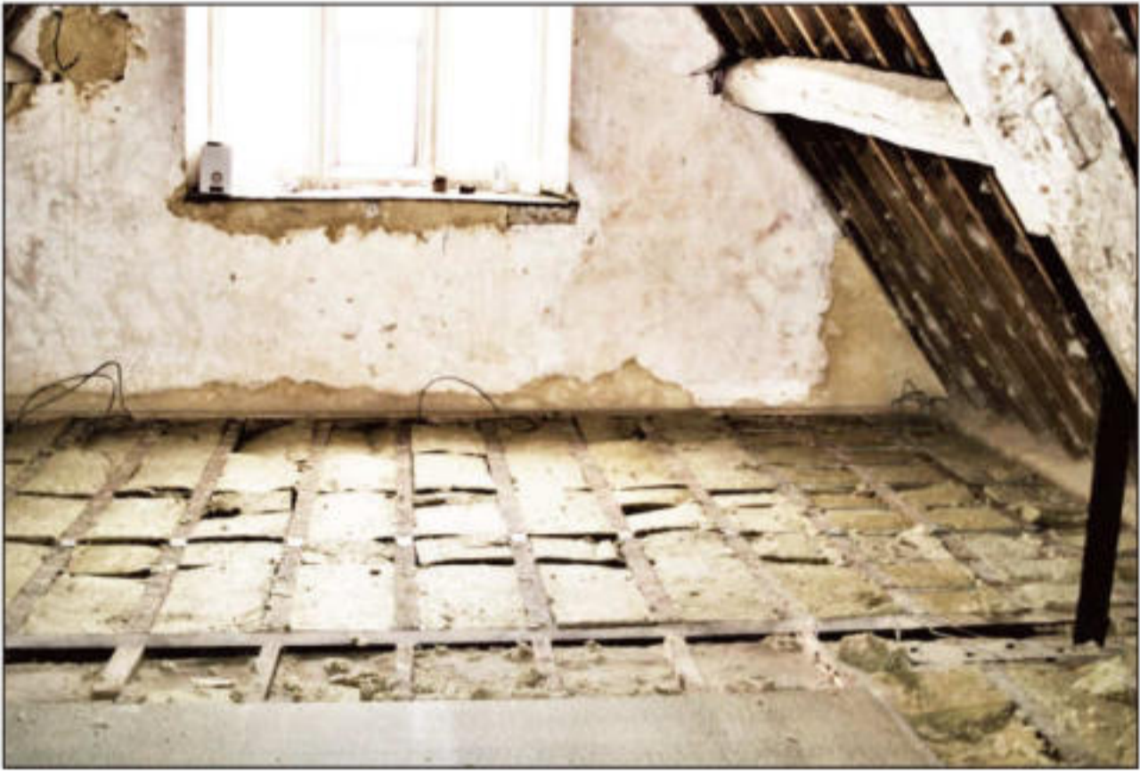
Sound Insulation to floor
