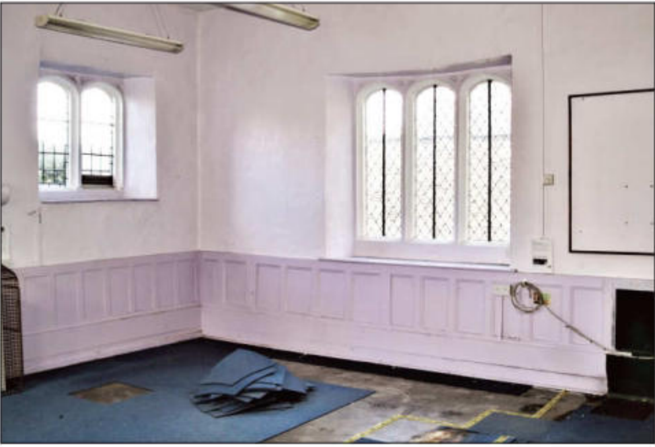
Library before work began
