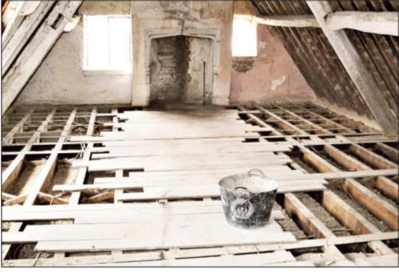
First floor boards removed
