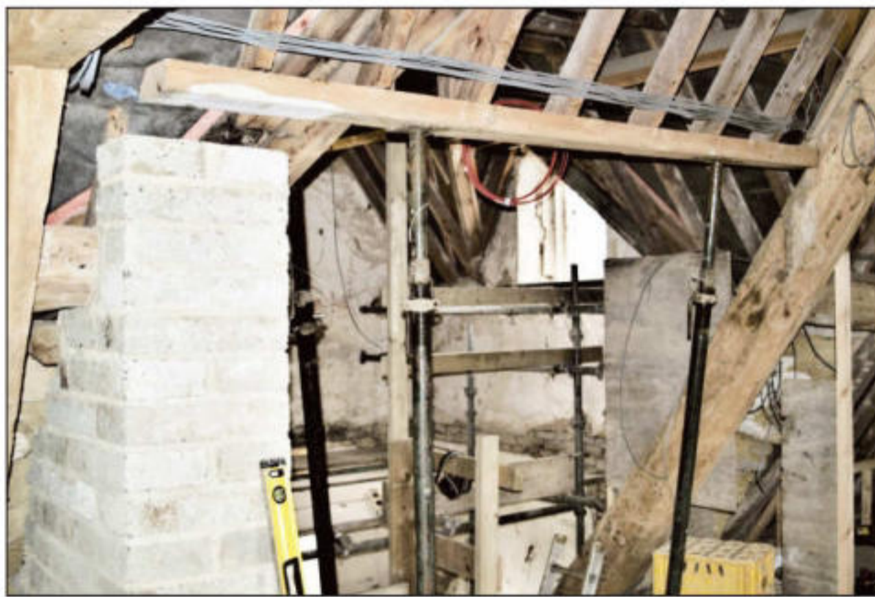
Altering beam for headroom
