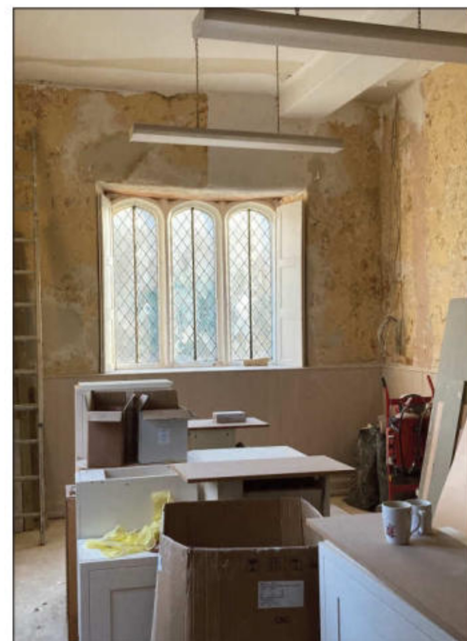
Vesey Room walls after stripping paper
