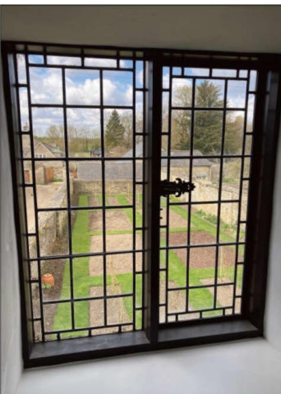
Upstairs window repaired
