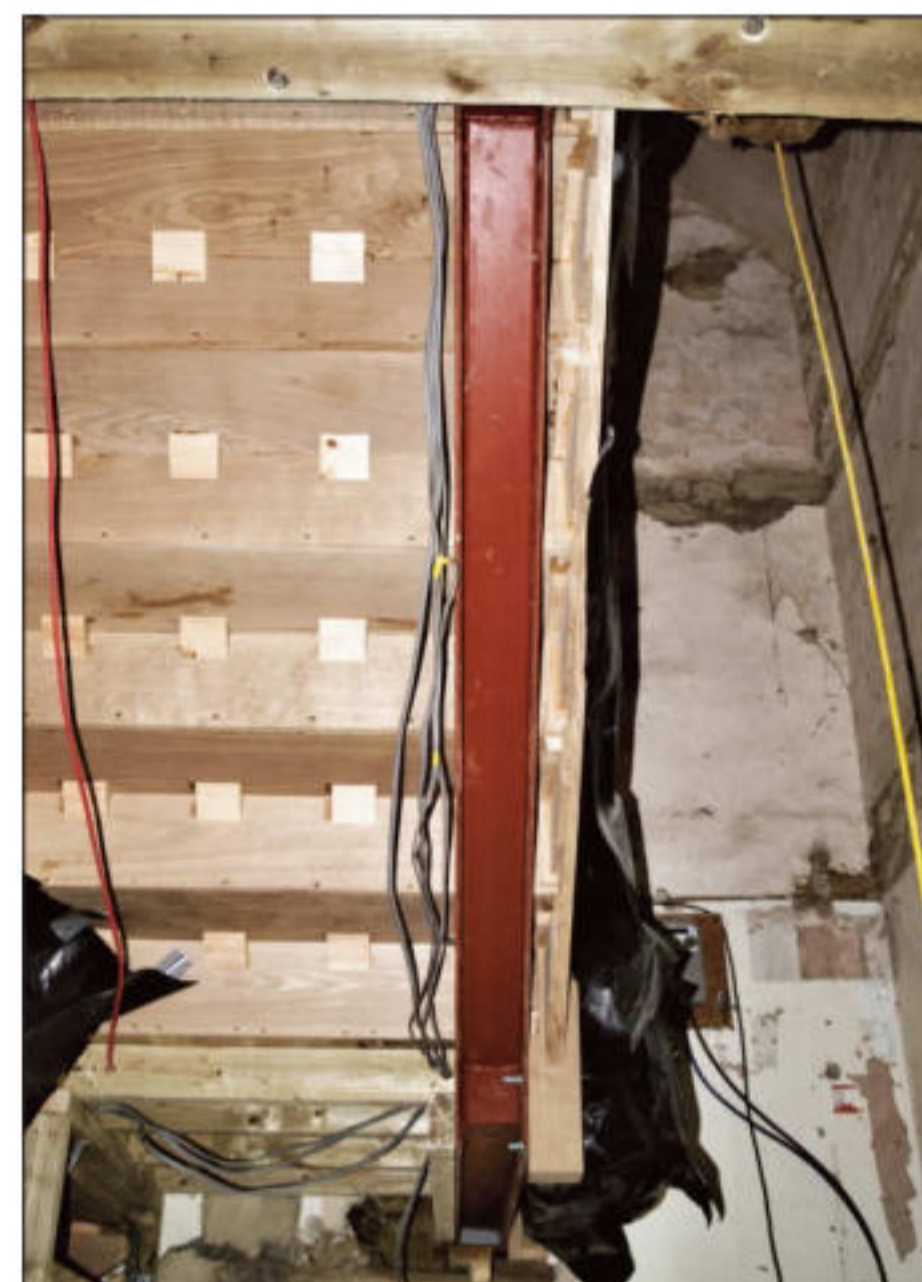
Steel beam with stairs
