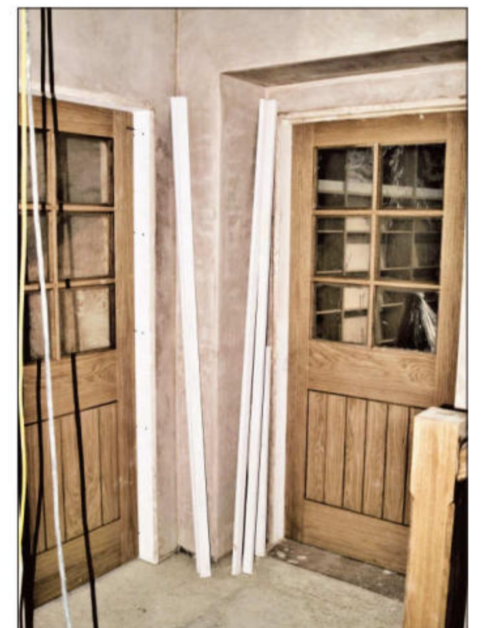
New doors fitted
