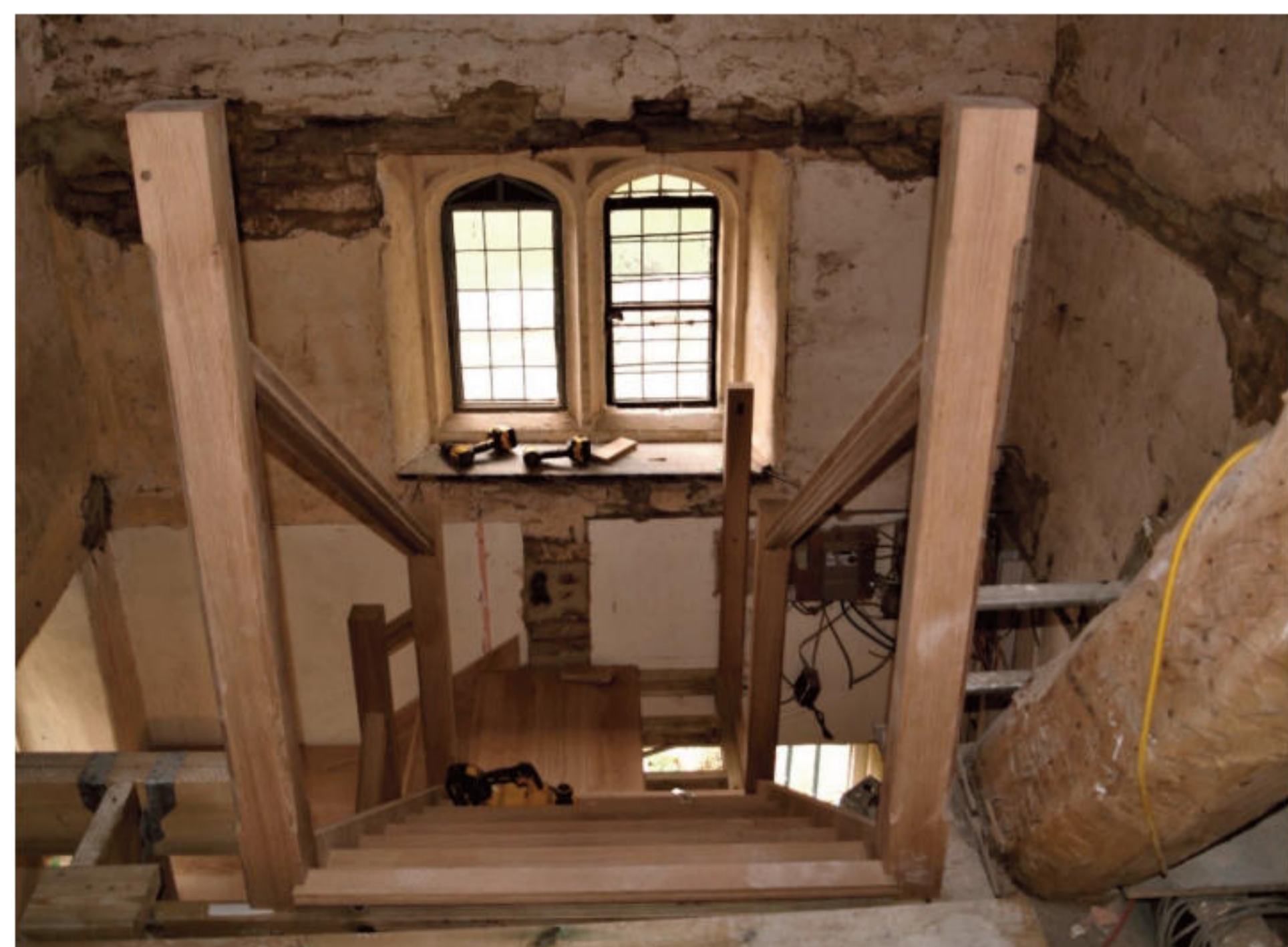
The new staircase under construction
