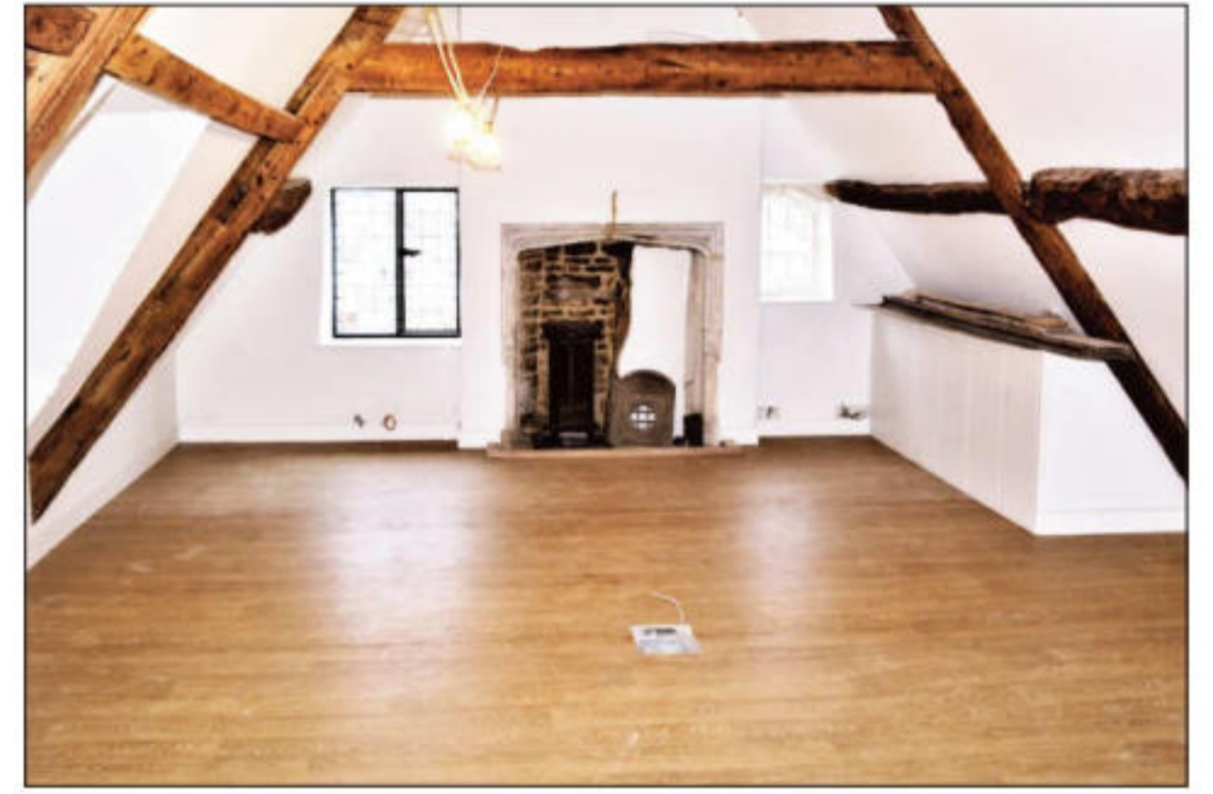
New floor laid
