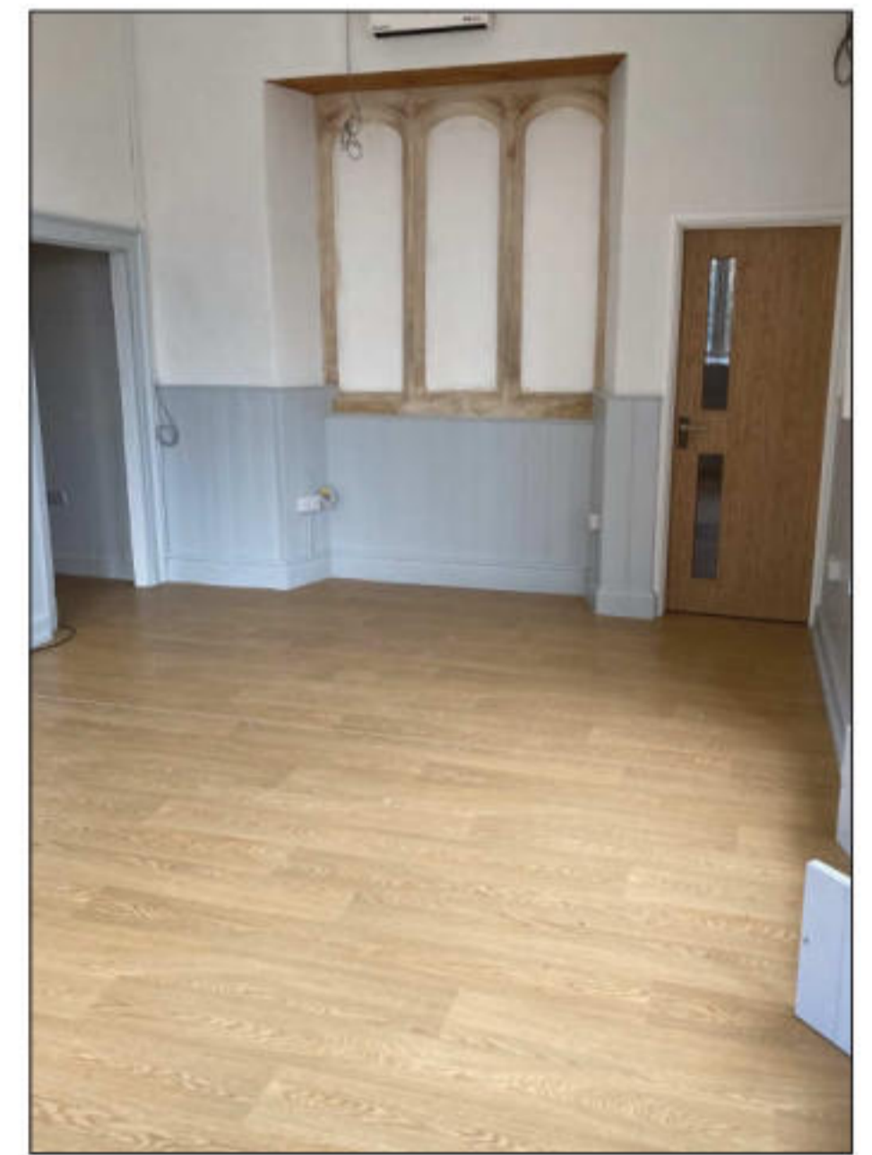
New floor Vesey Room
