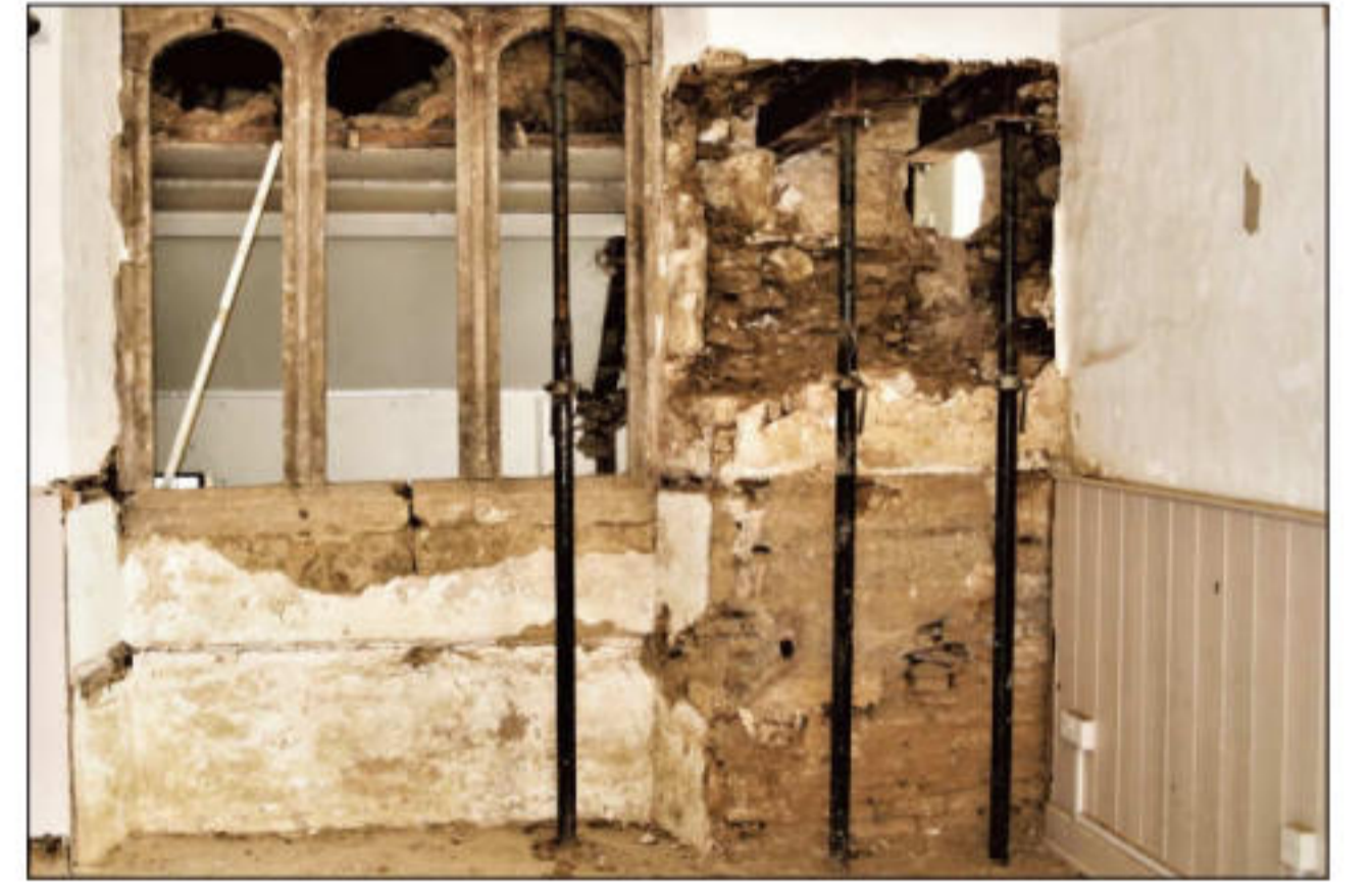
New doorway to kitchen
