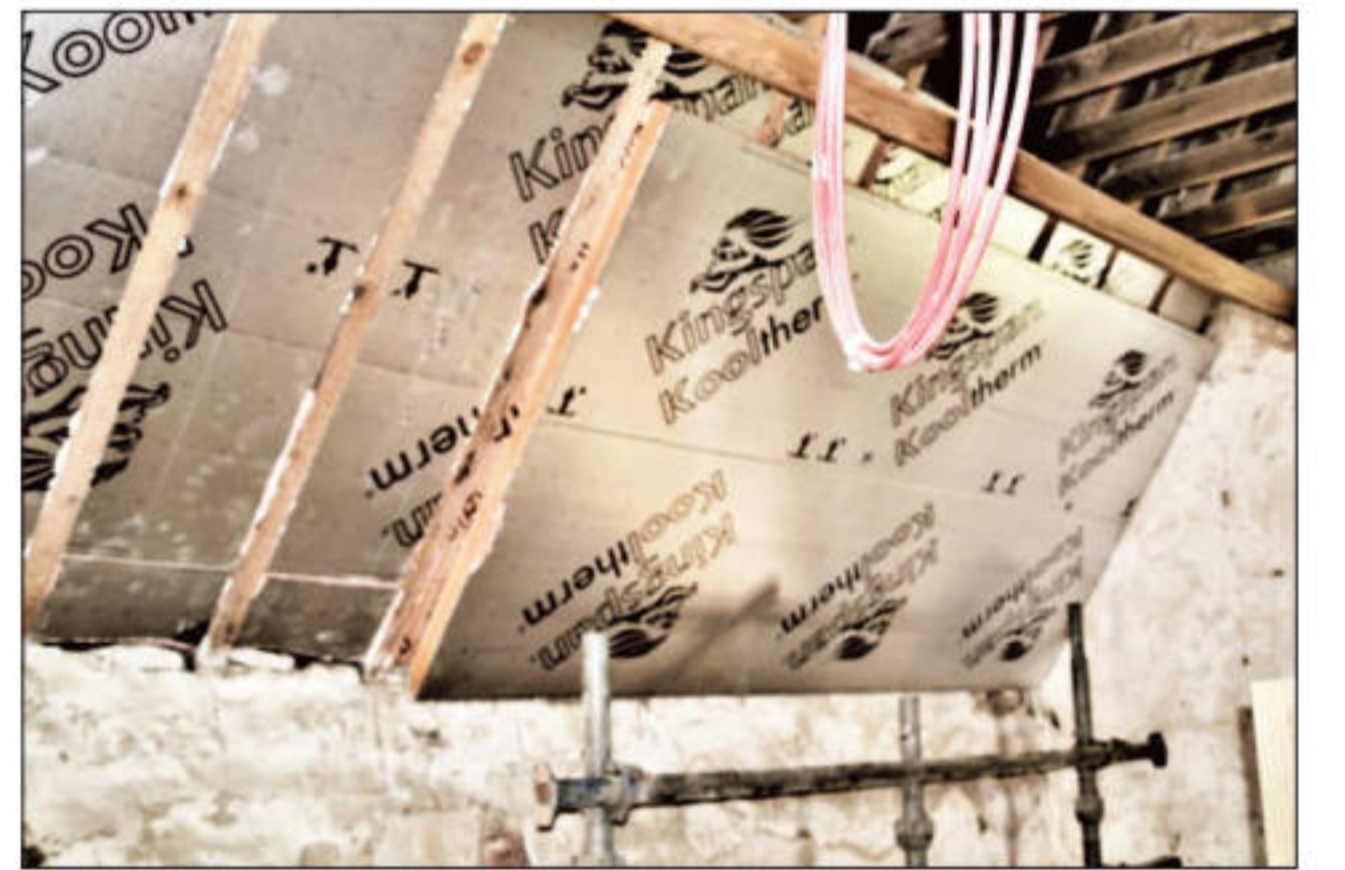
Roof Insulation - two Layers
