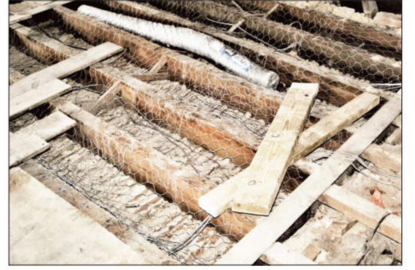
Mesh support for floor insulation
