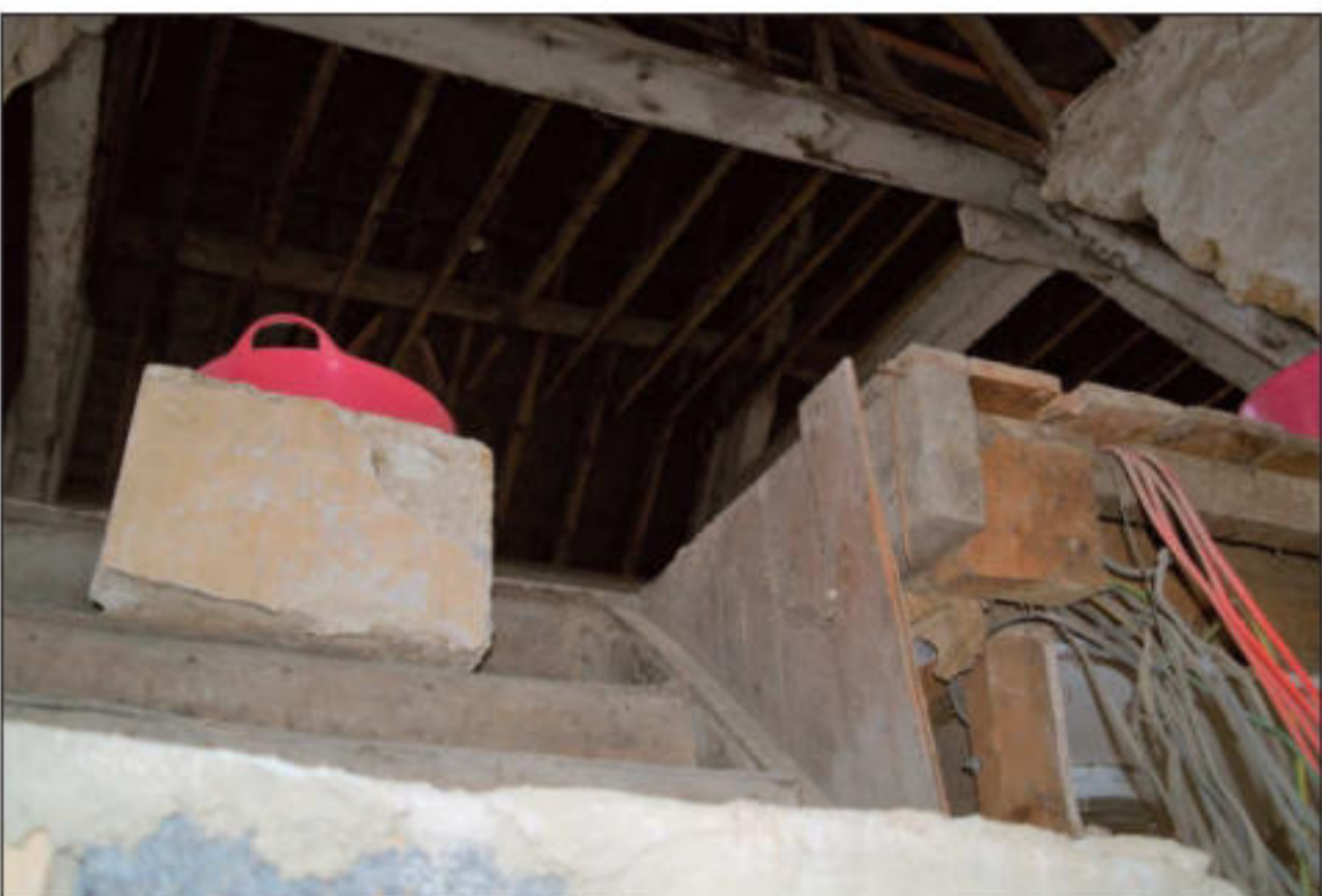
Demolition of the old stairs
