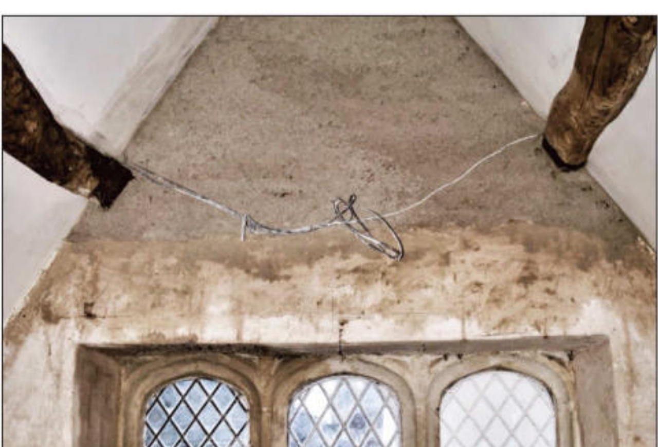
Lime plaster to gable
